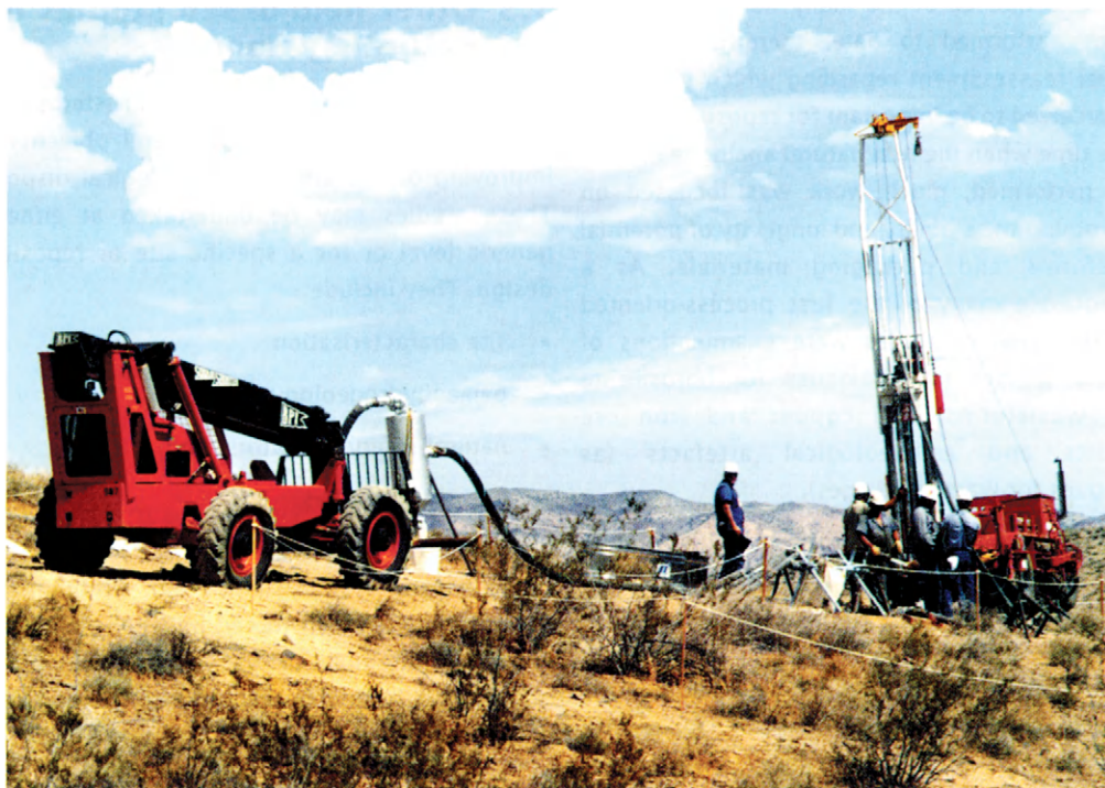
Figure 1.10. Site characterisation involves several techniques to learn about the subsurface rock and groundwater systems. In this picture boreholes are being drilled in the vicinity of the proposed US repository at Yucca Mountain, Nevada (see Section 2.3.1) to obtain samples of the rock from depth.
