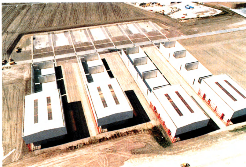
Figure 2.7: Photograph of the Centre de l'Aube surface repository for LLW in France. Wastes packaged in steel or concrete boxes will be placed in the large engineered compartments which are each 24 m long. When the repository is filled, the compartments will be sealed with a concrete 'lid' and the entire facility will be covered with an earth and clay cap, to form a small hill. Illustration courtesy of Nagra.
